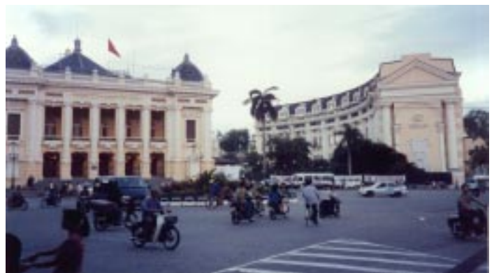
The new Hilton Hotel (right) in Hanoi complements the Opera House.
