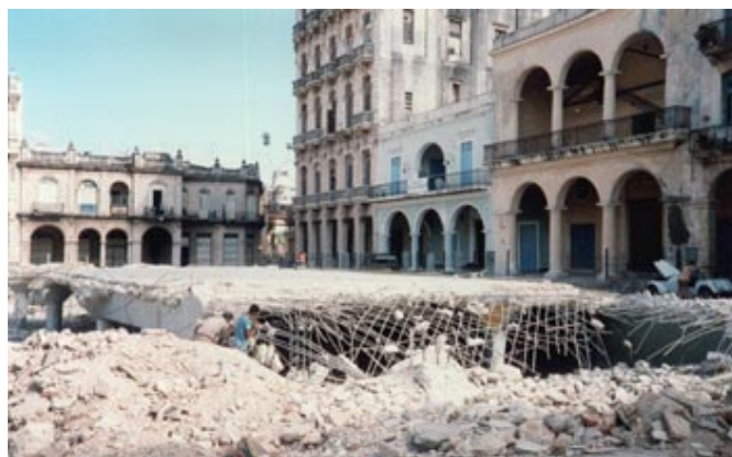
Reconstruction work in Old Havana, a designated UNESCO World Heritage Site
